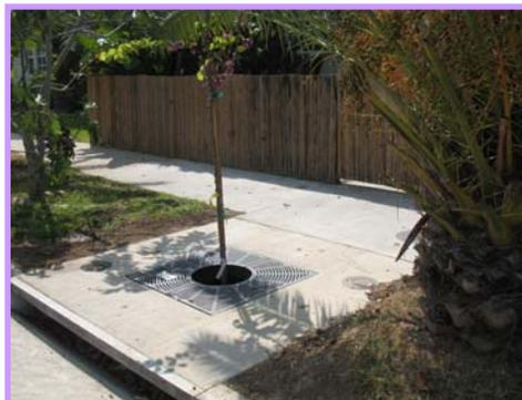
*Pictured Right: A filter unit is already in place to capture stormwater from the surrounding area.*
